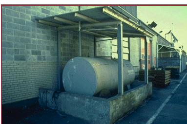
7 - Covered AST with secondary containment (above)
