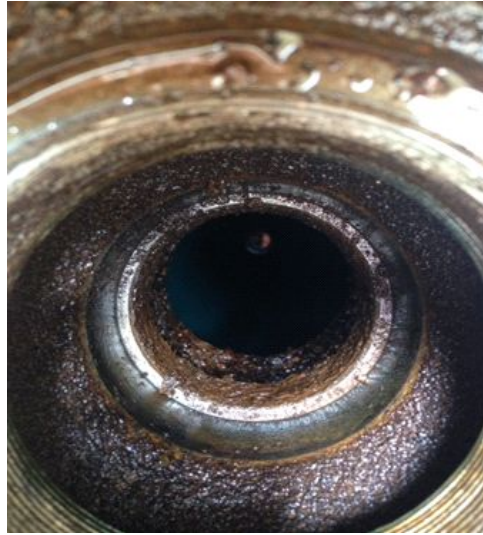
Figure 3: The suction tube attachment to the sump. This is the highest point in the system with relatively little or no contact with fuel. This piece has no exposure to outside environment.
